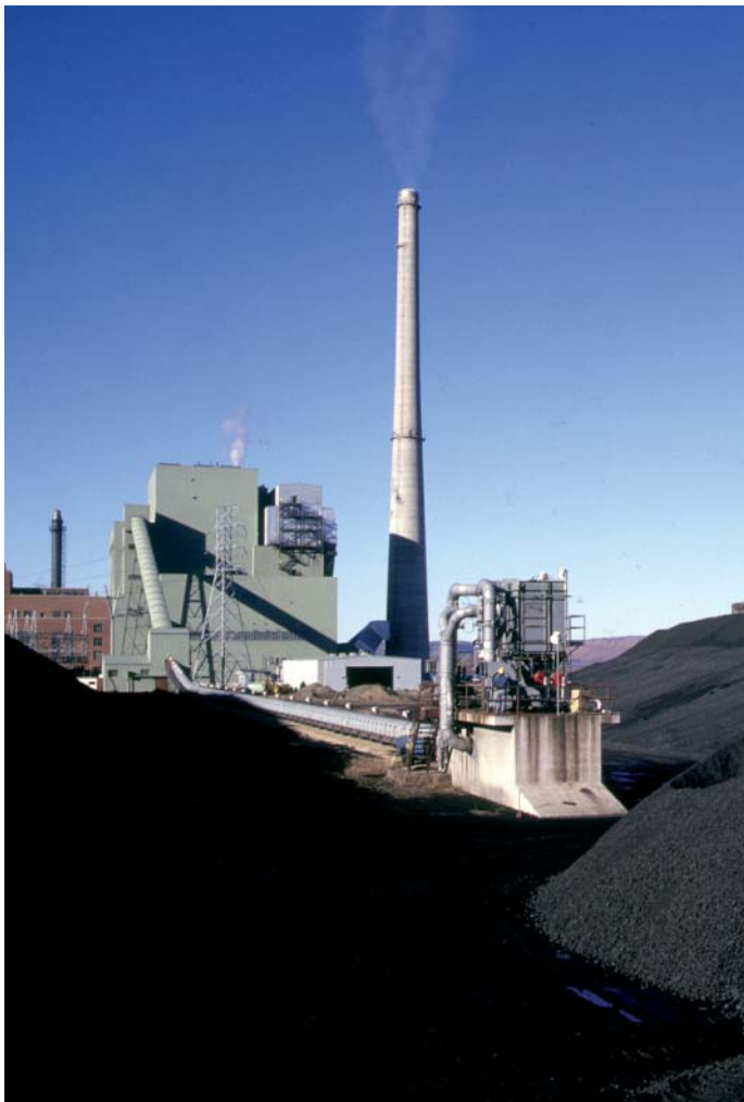
Our experience and expertise allows us to develop and implement a combustion improvement project from start to finish.
